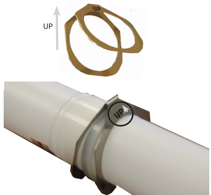
FIGURE 6-4 - (NATALINI) CLAMP EXAMPLE
